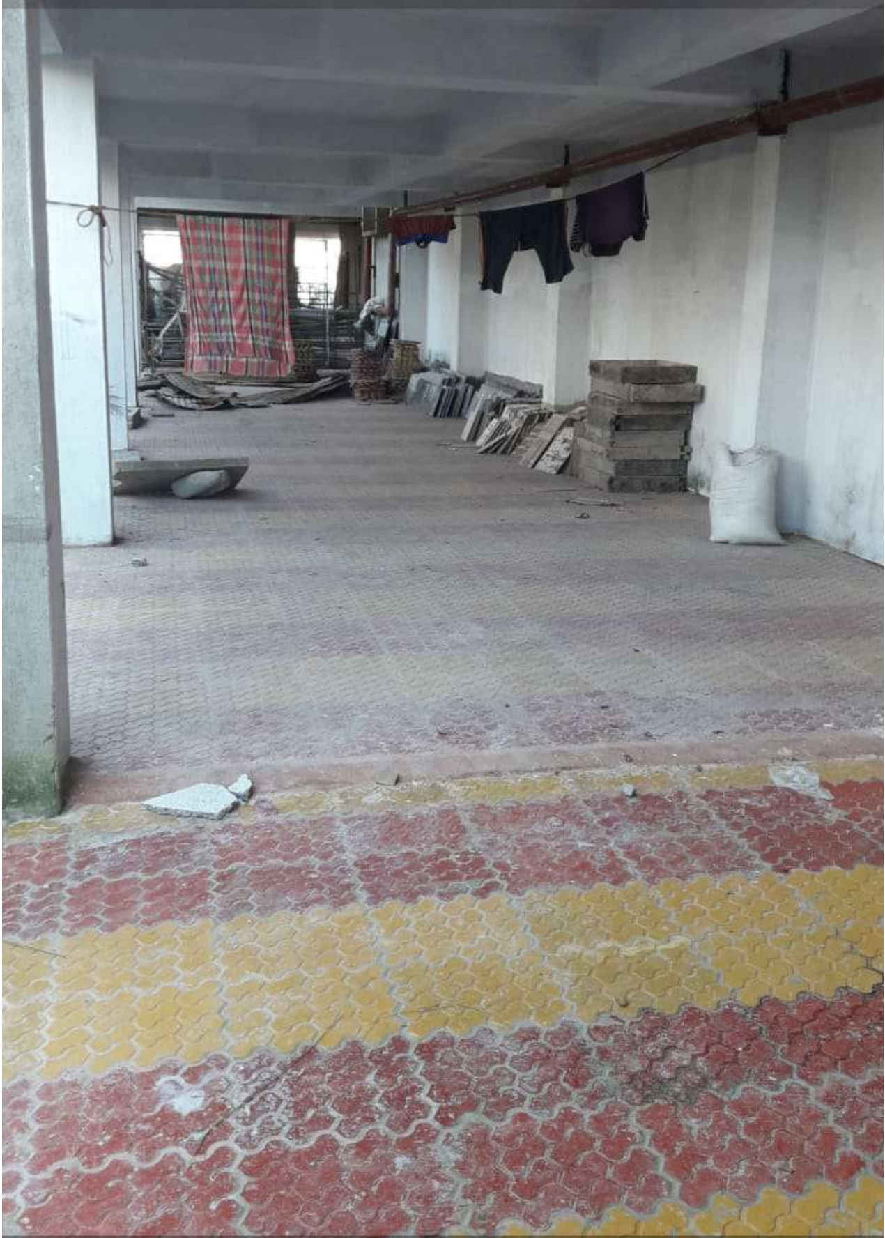
Block- D, parking/Basement
